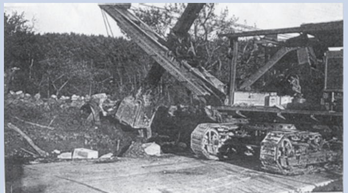
Our Old Roads: Route 101 in Dublin has a concrete road base that was installed in the late 1920s. The current traffic-calming project had to remove some of the base to lower the hill above the fire station. This photo shows the concrete being put down and a Mike Mulligan-type steam shovel doing the work.
