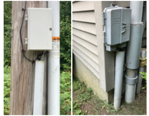
Two examples of buried conduit at pole and home.
