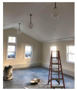
Work on the new DubHub addition was projected to be done by Christmas. Shown in this photo walls and trim painted, new light fixtures and track lighting. The new flooring is a rubber product – durable with "give." The pattern blends with the warm white paint selected for the walls.
