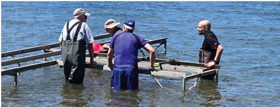
Volunteers help install the dock at the DWCC beach.
